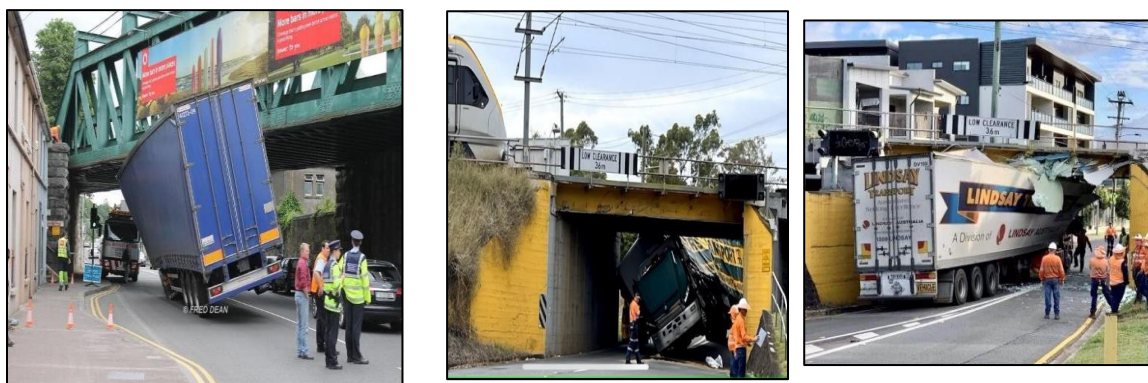
FIGURE 3. References image of railway bridge tunnel damage identification & Protection
